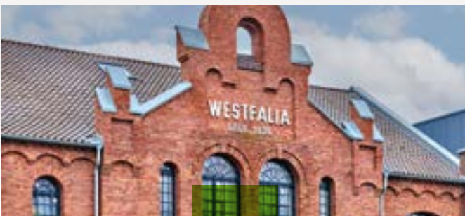
Mine Westfalia, Lünen
