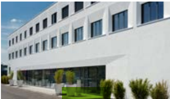
Administration building, Jettingen-Scheppach
