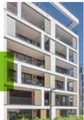
Balcony protection, apartment block
