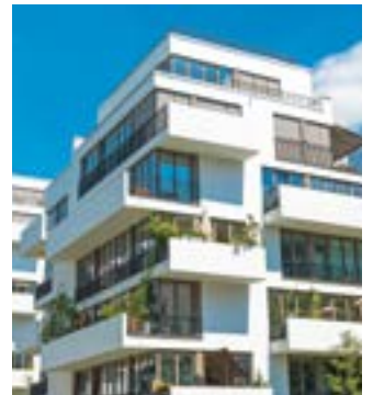
Balcony protection, apartment block
