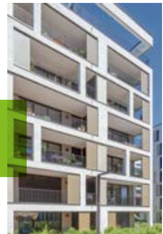
Balcony protection, apartment block
